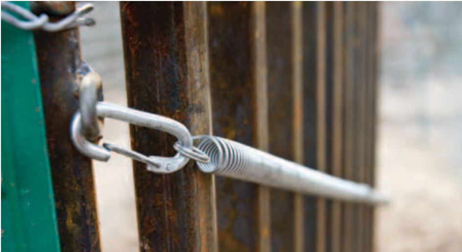
A fastener used to connect the spring to a link of chain welded on a spring door
