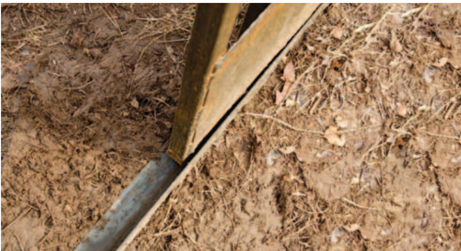
Frame all doors with angle iron to prevent hogs from pulling them open from the inside.
